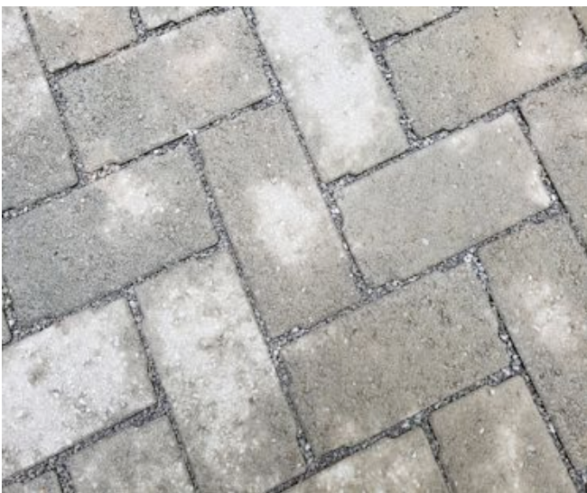
Figure 3 PICP joints properly filled
